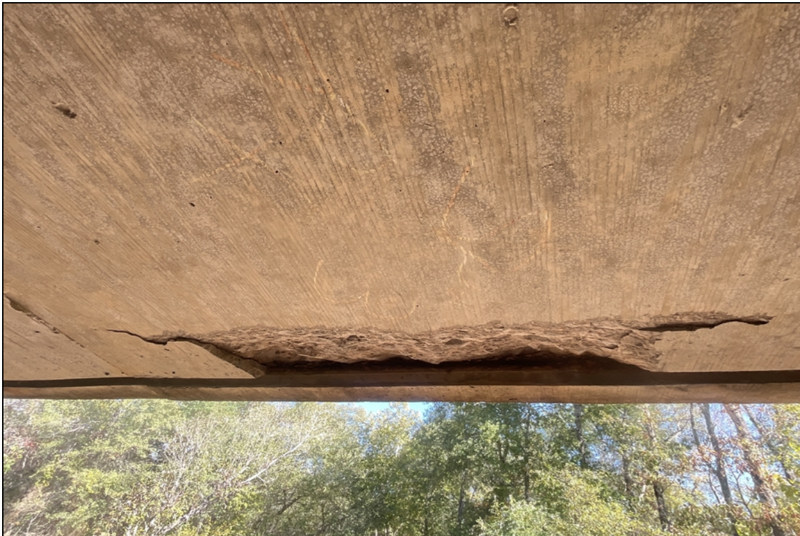
Spall with exposed reinforcing steel in the right drip groove of span # 3.
