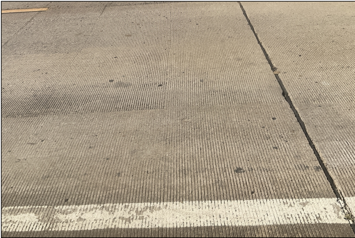
Longitudinal cracking in the driving surface of span # 2.
