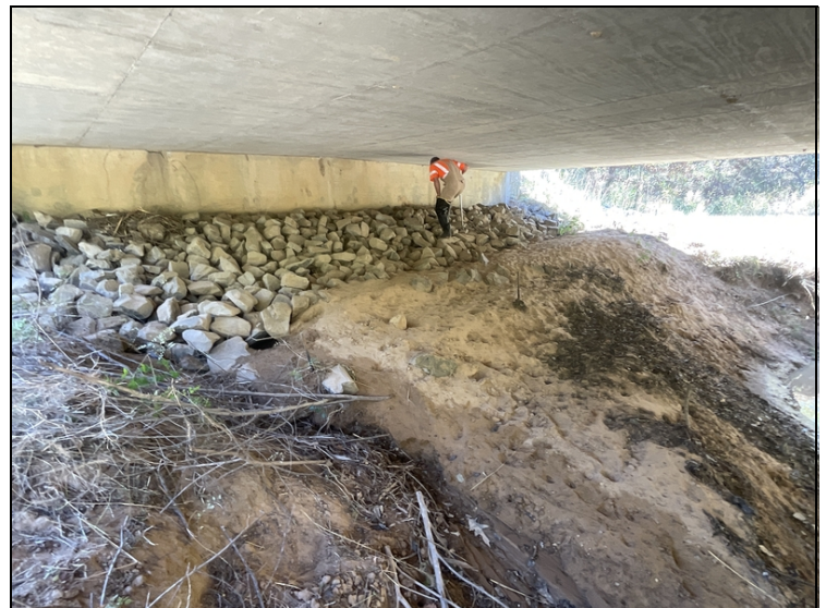
Minor rip rap displacement. South abutment.
