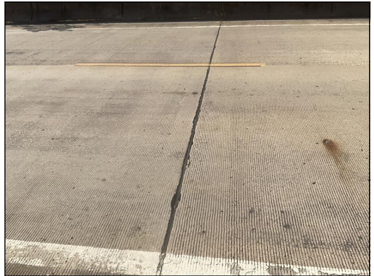
Expansion joint seal over Bent # 4. Leakage.
