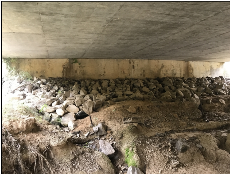
South embankment-Erosion.
