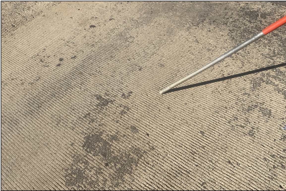
Hairline longitudinal cracks in the driving surface of the slab. Span # 4.
