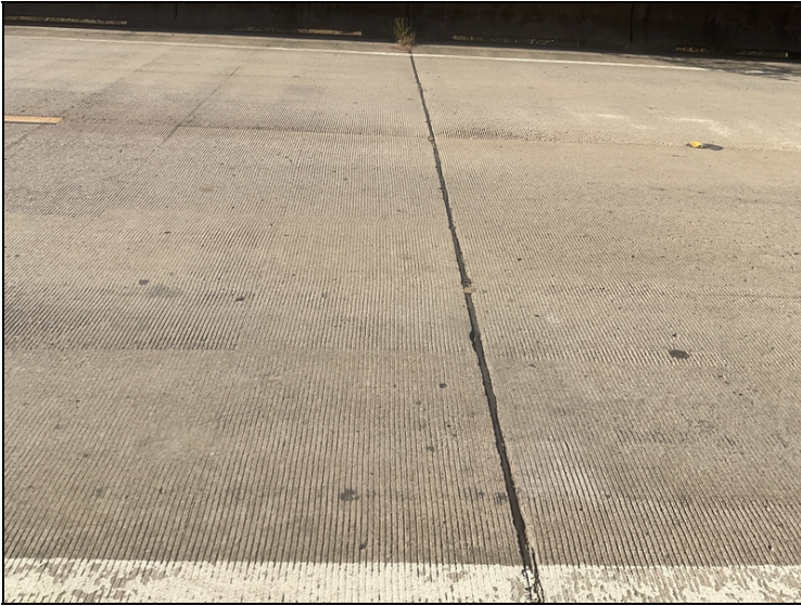
Leaking expansion joint sealant over bent # 3.
