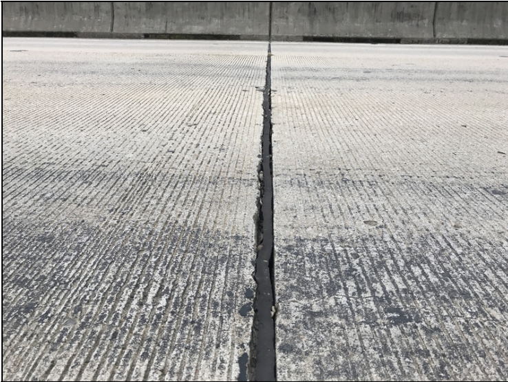
Expansion joint over bent # 3-Adhesion failure.
