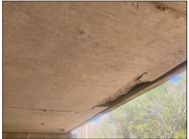
Span # 3. Spall with exposed reinforcing steel in the Right drip groove.
