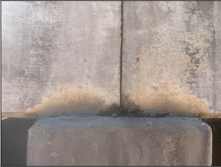
Minor concrete deterioration in edge of slab over Bent # 4 Right.
