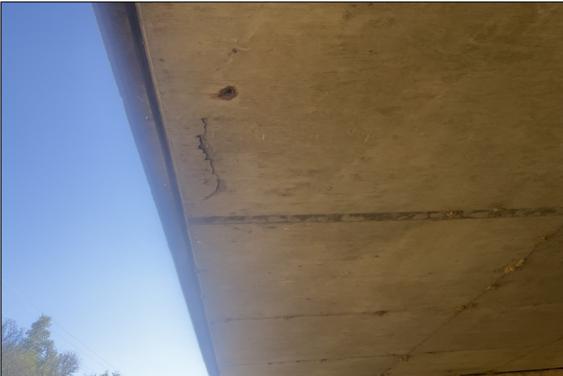
Span # 2. Right. Delaminated area along the drip groove.
