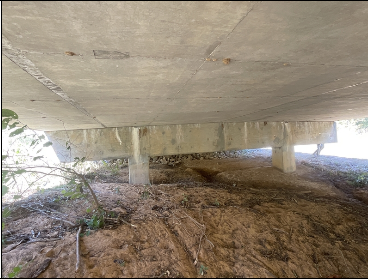
Leakage on bent # 4 cap.
