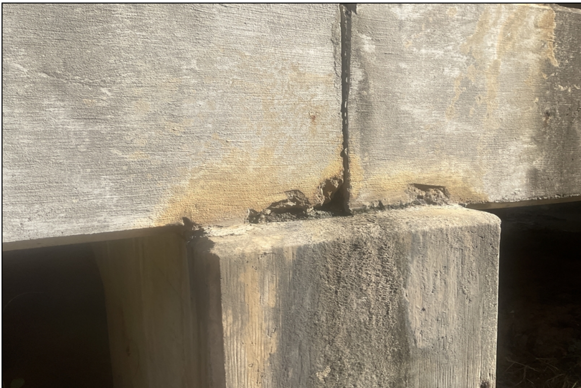
Left edge of spans # 3 & 4 over Bent # 4. Concrete deterioration.
