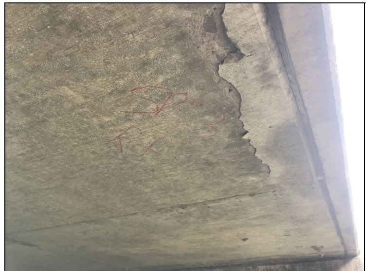
The undersurface of the slab has delaminated areas along the drip groove on the right side in span # 3.
