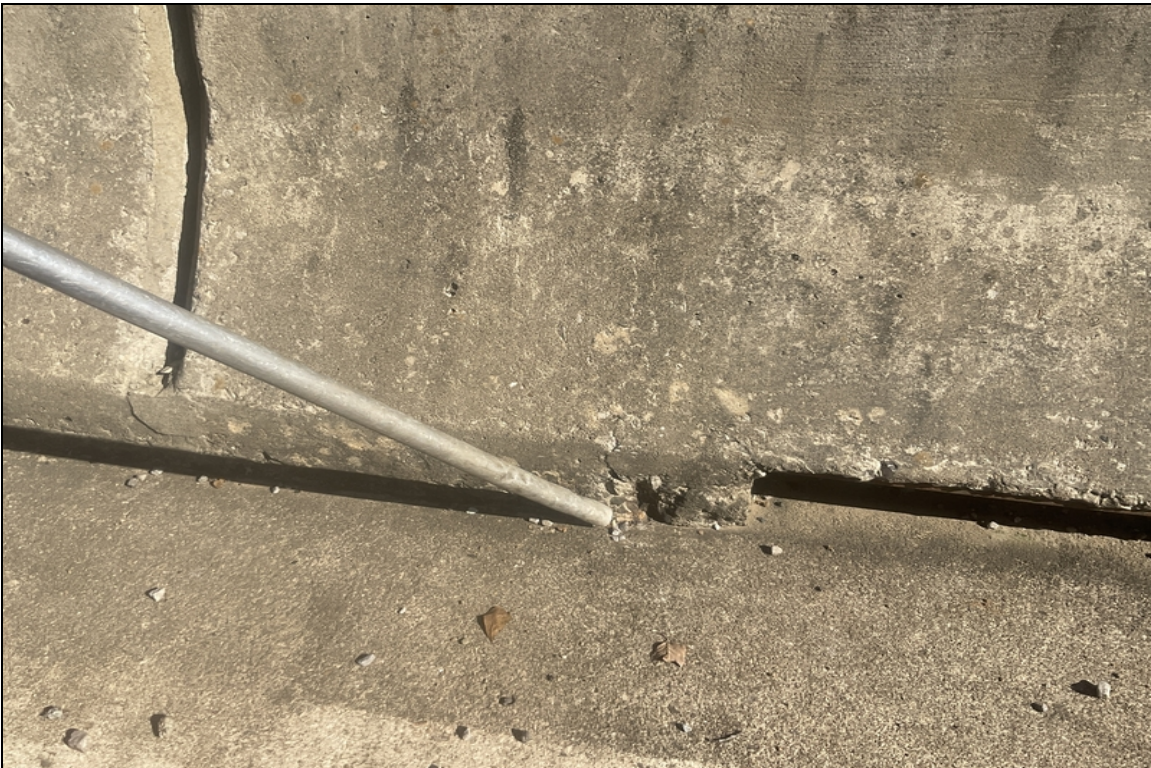
Spalls with exposed reinforcing steel at the base of concrete parapet. Span # 3. Right.
