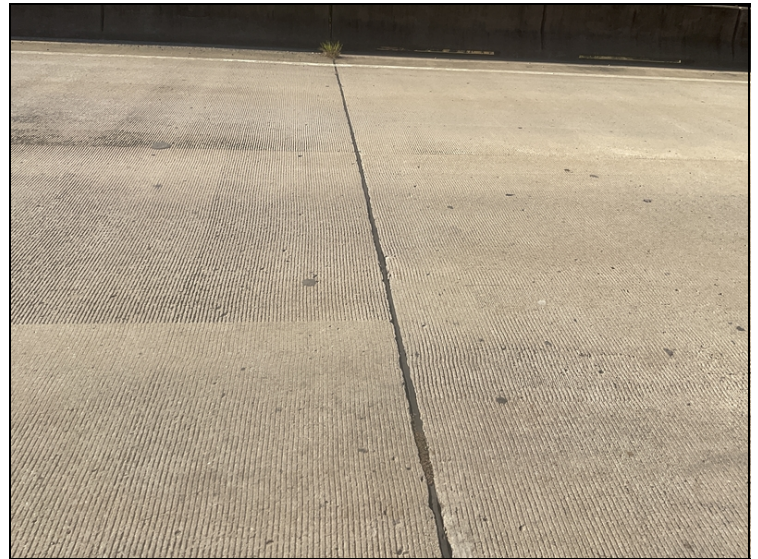
Leaking expansion joint sealant over bent # 2.
