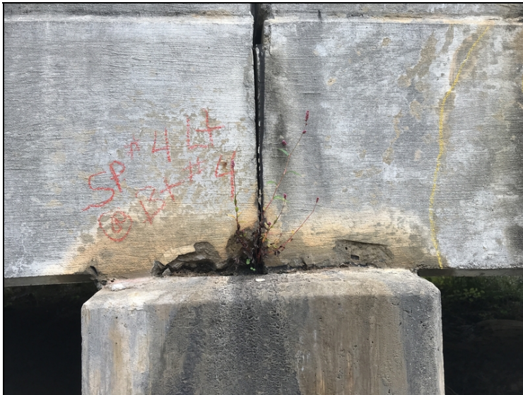
Span # 4, left-Shallow spalls in ends of slab on exterior sides over intermediate bents.
