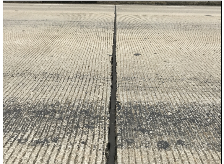
Bent # 2 expansion joint-Adhesion failure.
